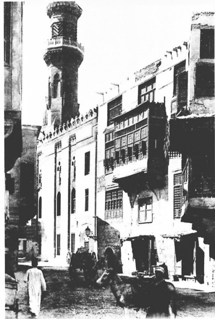
CAIRO - Street Showing Harem Windows. - II.
