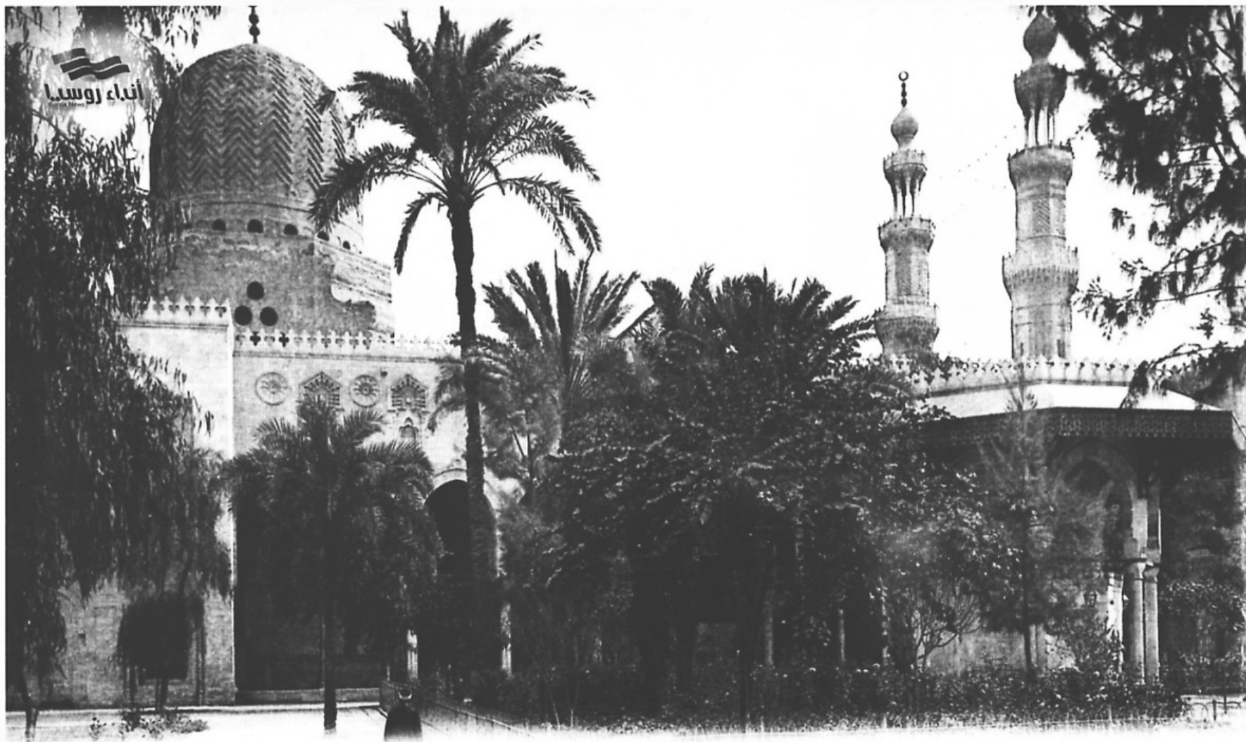
73 CAIRO. — Courtyard Mosque Moerirt. — 11
