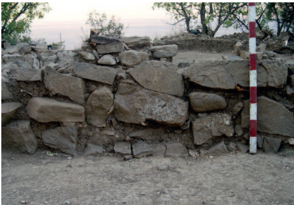
Рис. 1.21. Северный вход в храм. Закладка проёма в третьем строительном периоде. Вид с юго-востока. Fig. 1.21. Northern entrance to the church, closing of the doorway between northern and southern parts of the church in the third building period, view from southeast.
